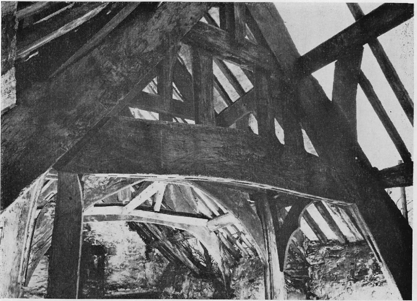
FIG. 12. Truss D. From Service Room
